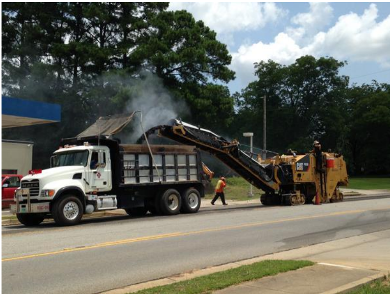
Resurfacing of Robert Toombs Avenue in downtown Washington, GA
