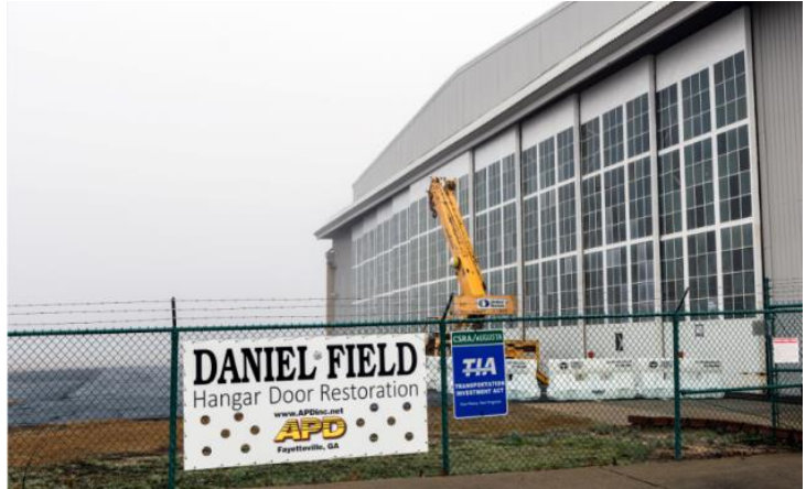
Daniel Field Hangar Door Restoration
