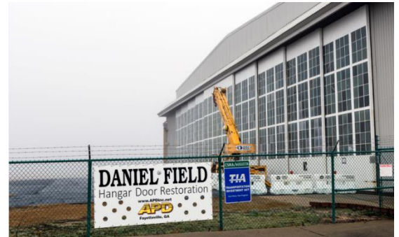
Daniel Field Hangar Door Restoration
