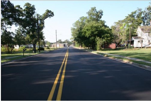
Resurfaced Brumby Street in Reidsville, GA
