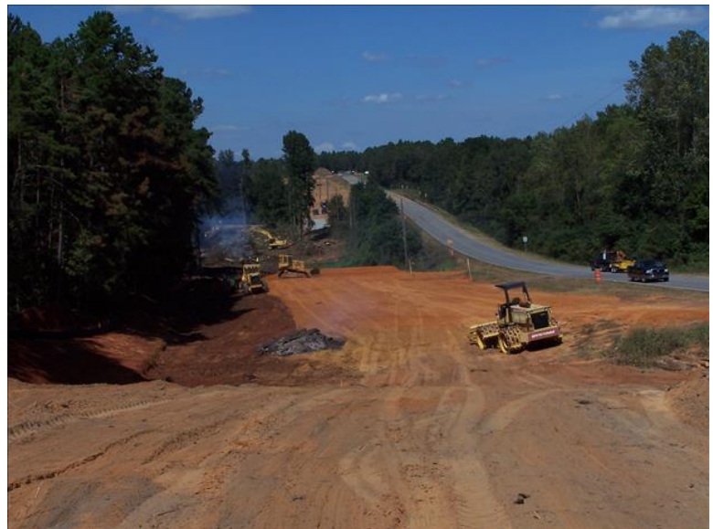
Construction along State Route 1 / US 27
