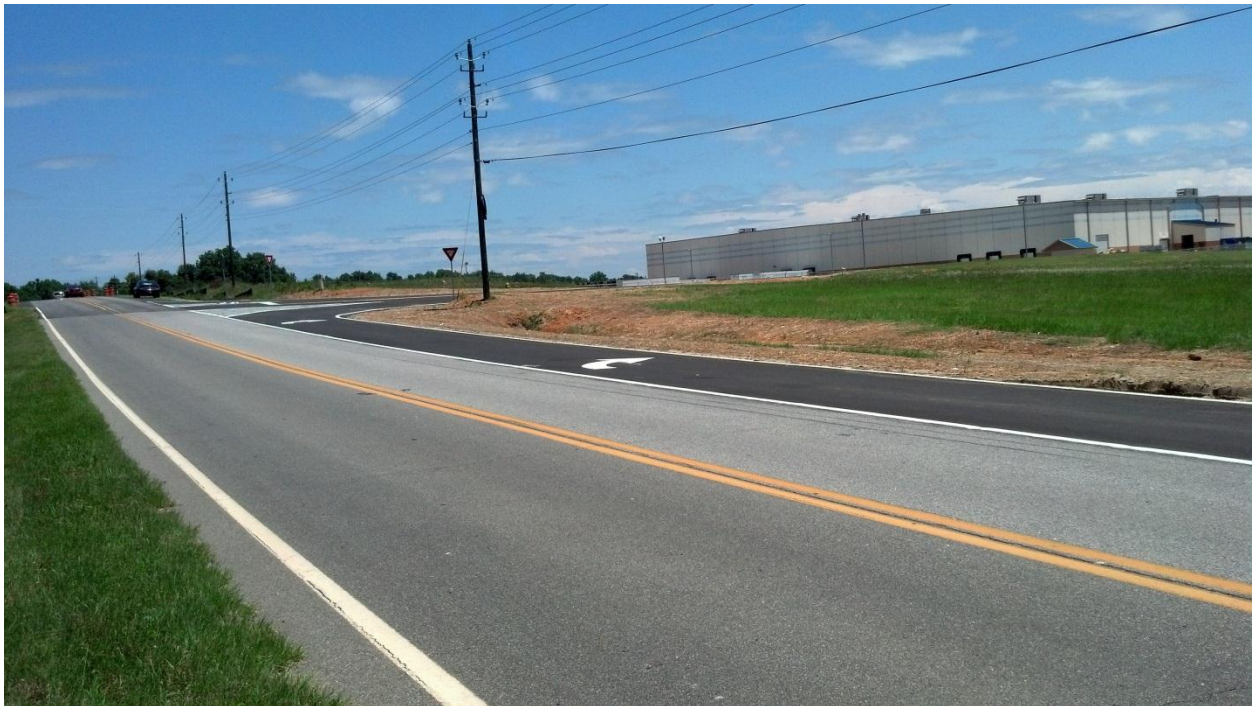
New turn lane on S.R. 130 Toombs County
